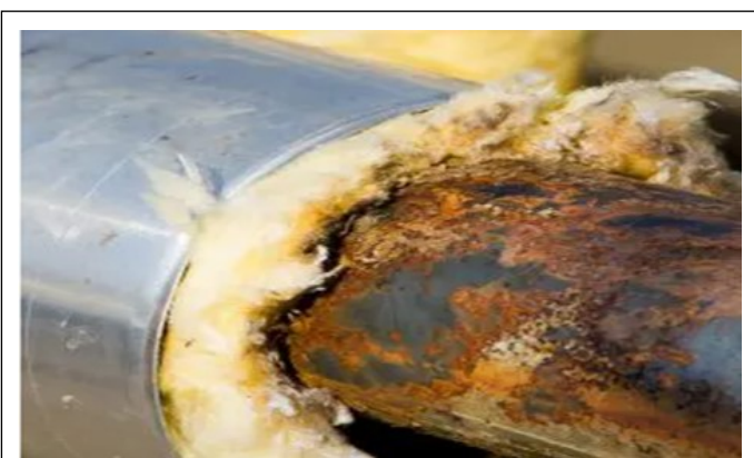
Fig.5. visual test method for corrosion under insulation
